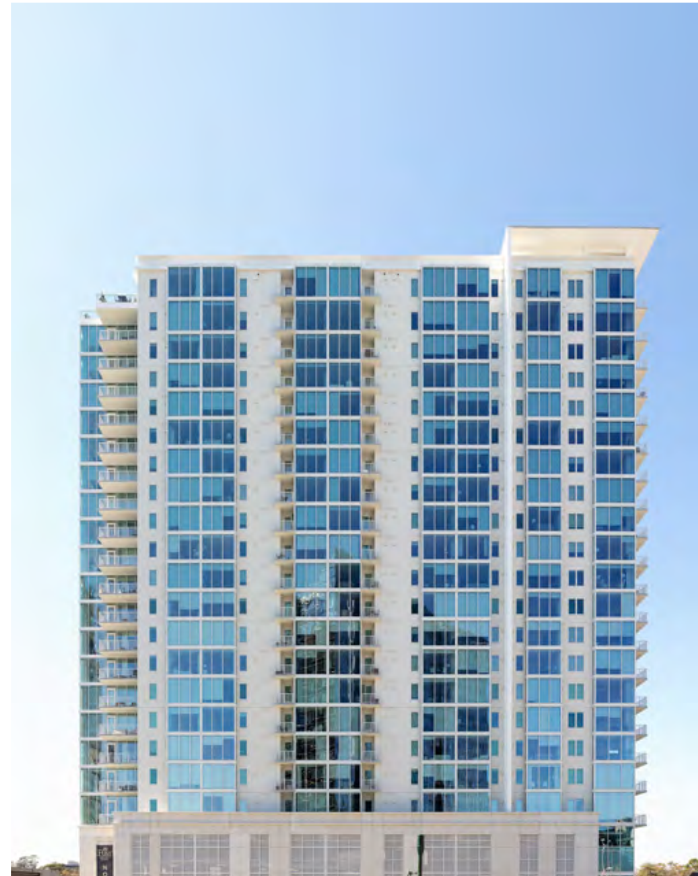
MAA Lenox | Atlanta, GA | NGBS-certified MAA Lenox received consecutive ENERGY STAR certifications in 2021 and 2022.
