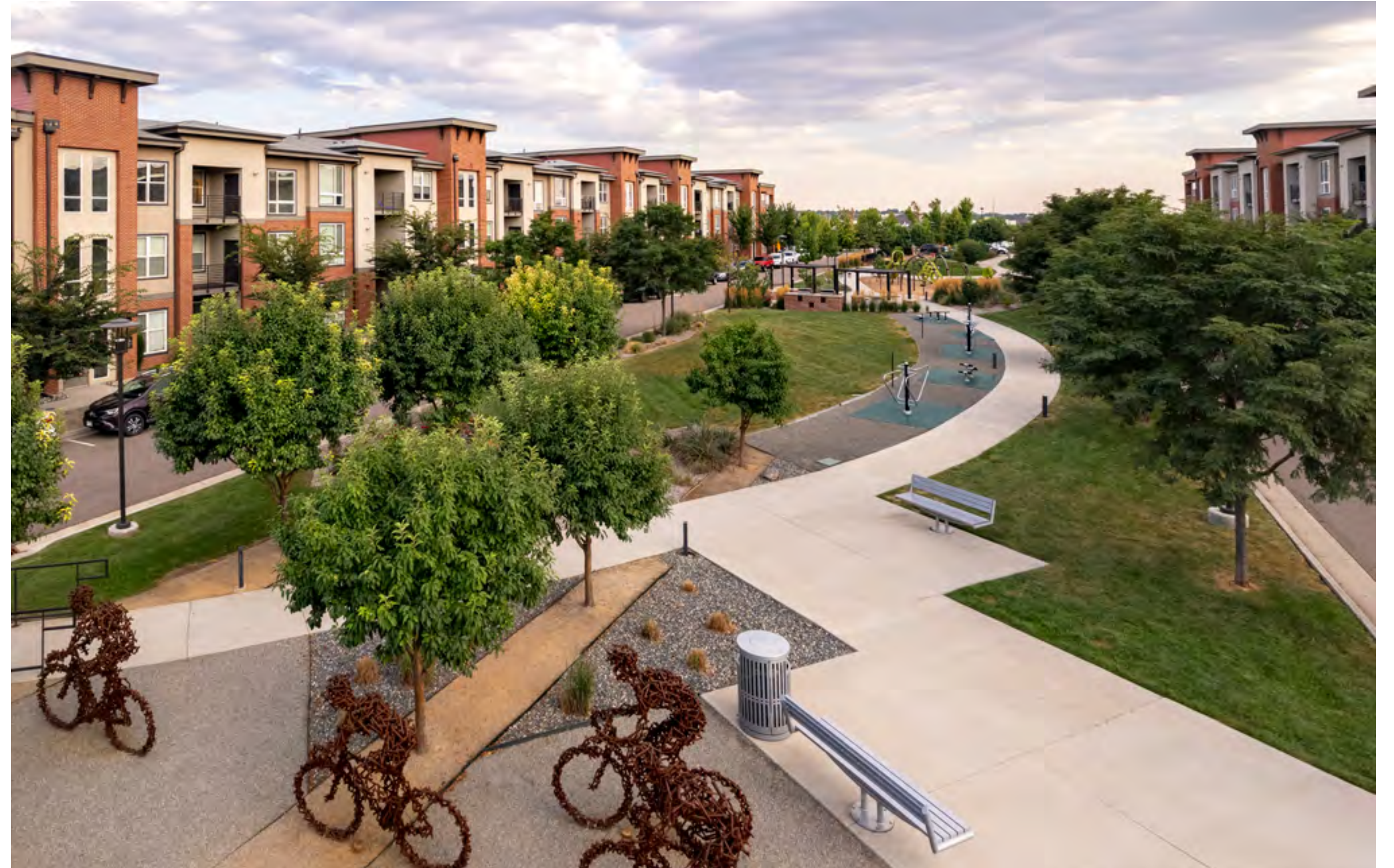
MAA Promenade | Denver, CO | An energy audit and subsequent LED light conversion project at MAA Promenade improved the overall energy savings potential for residents.
